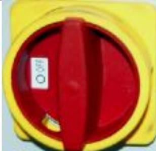
A red emergency stop button with a yellow border. The button has a white label with 'OFF' written on it.                                           | Absperrbarer Netztrennschalter an der Unterseite des Schaltkastens                                                                                      |
